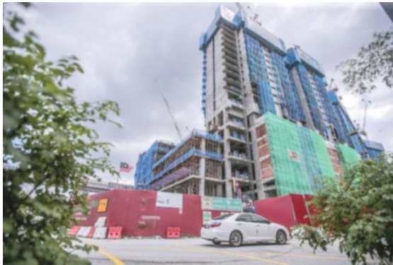
A general view of the Pavilion Damansara Heights construction site in Kuala Lumpur. (Pic: Hari Anggara)
